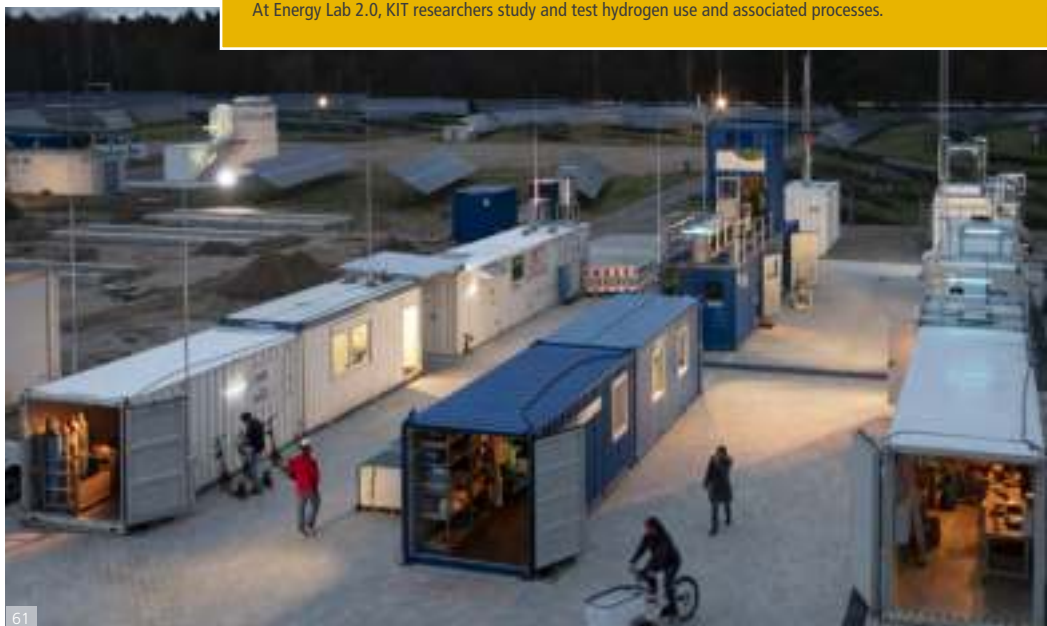
At Energy Lab 2.0, KIT researchers study and test hydrogen use and associated processes.
