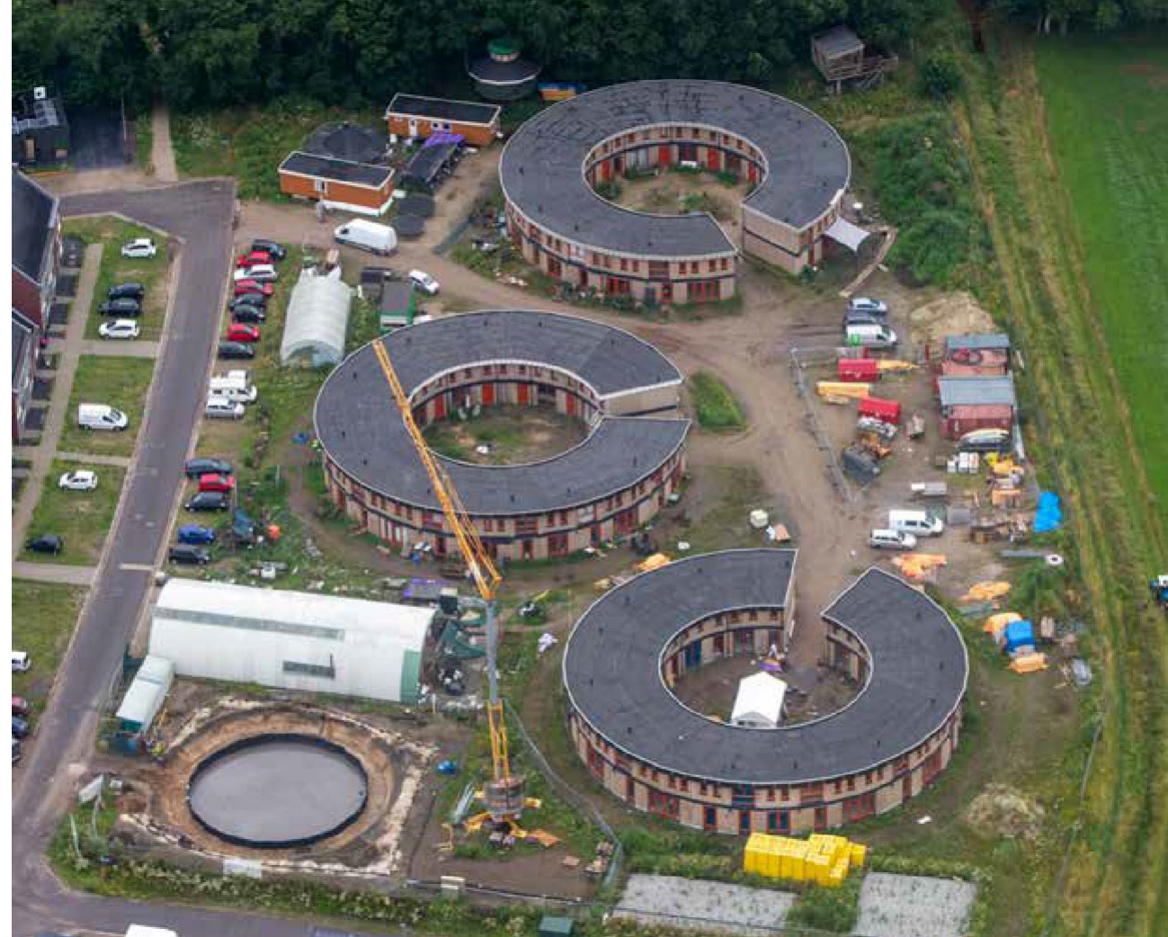
Ecovillage Boekel under construction. The construction of the heat battery (bottom left) has just started, it will be put into use at the end of 2022.
